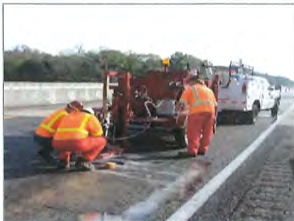
Figure 2: Photo of Standard Penetration Testing (SPT)
