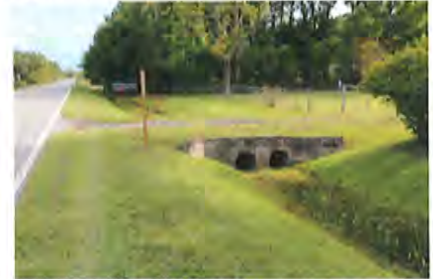
Figure 16: Side Drain Hazard in Clear Zone
