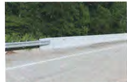
Figure 18: Existing Substandard Guardrail Connection to Bridge Barrier Wall
